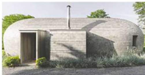
Rounded buildings use up to 20 per cent less material than rectangular structures, make breezes move more efficiently and dissipate sound waves.
