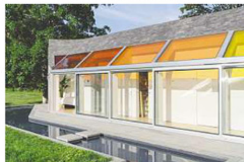
The reflecting pool/cistern collects rain run-off for garden irrigation.
